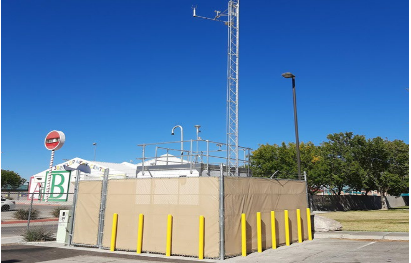
Figure 3-16. Walnut Community Center
